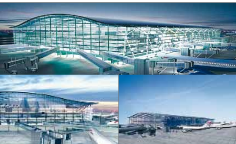
Terminal 5, Heathrow Airport, London
